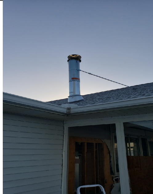
4. Above roofline portion of the chimney, as seen from ground level
