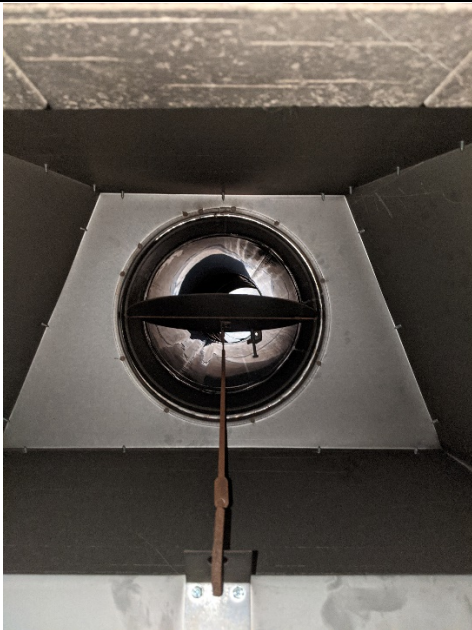
3. Fireplace Damper, looking up the chimney
