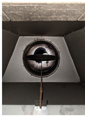
3. Fireplace Damper, looking up the chimney
